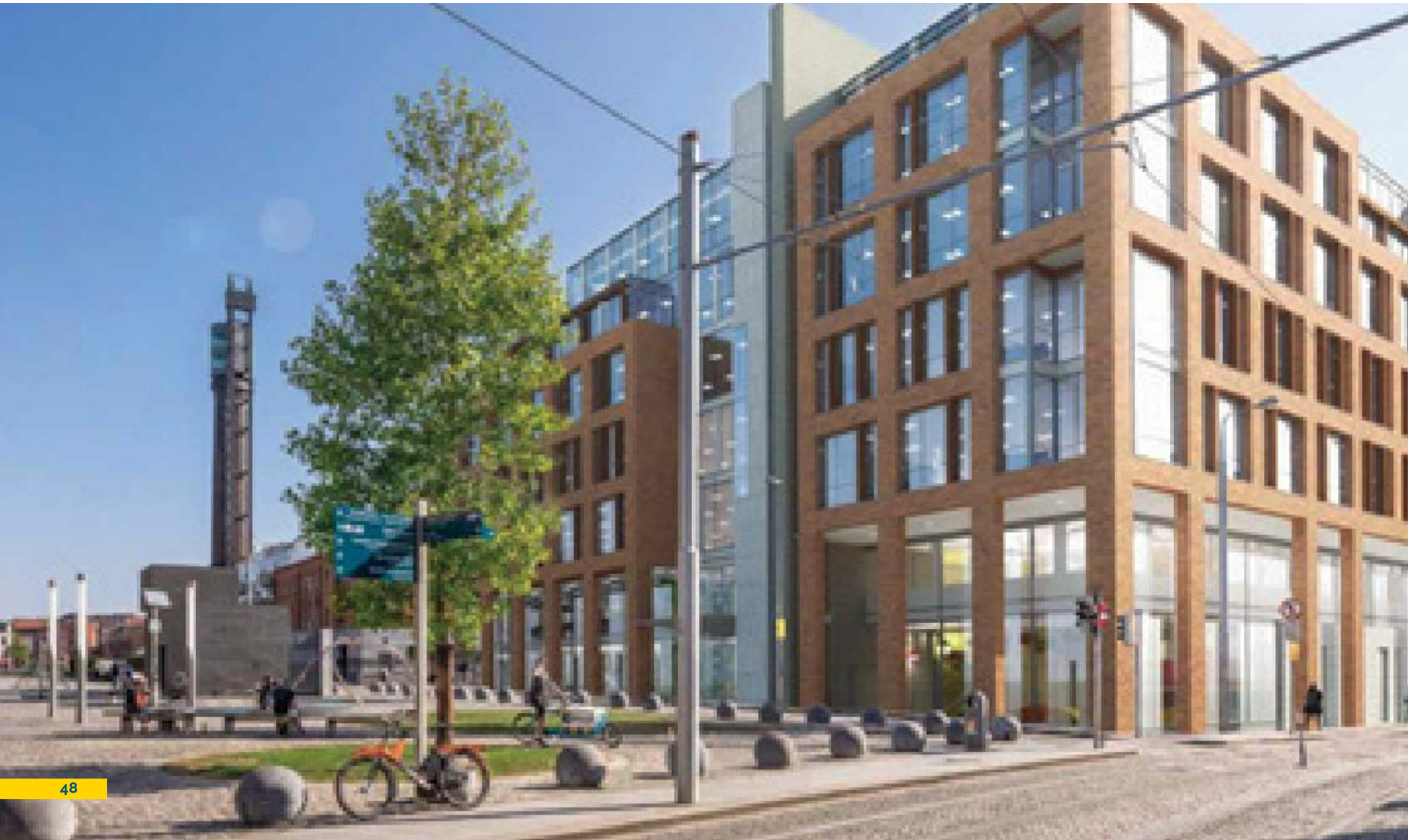
Figure 23: Mixed Use Commercial Project Smithfield, Co. Dublin
