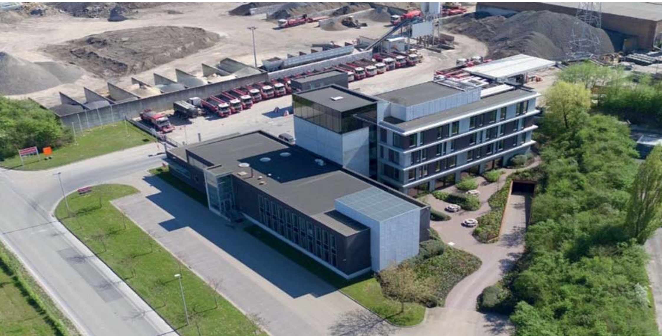
Figure 4: Stadsbader office building
