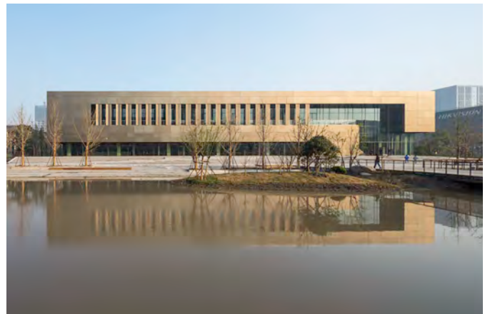
Research and Development Center Huawei, Huangzhou (China)
